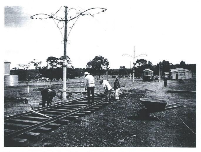
Major repairs to the south end of the main-line continue. The hard and laborious amount of work being undertaken is evident and a credit to those involved. Once the resleepering is finished, it will require lifting and packing with ballast. Until the work is completed, tram No 427 will remain at the terminus.
