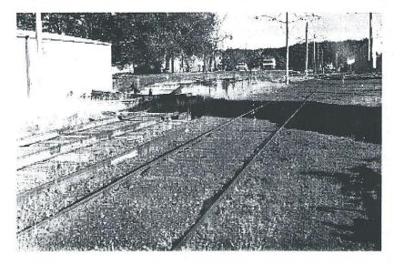
Seen here is the main-line at the depot junction after the repairs were undertaken to install six tie-bars to bring the track back into correct gauge. To the left can be seen the current southern end of the new (future double siding track) constructed as part of the trackwork Vehicle the Maintenance Building. As that new track is laid in tramway rail, it has been set slightly lower so that the railhead is level with the railway type rail in the current main-line.
